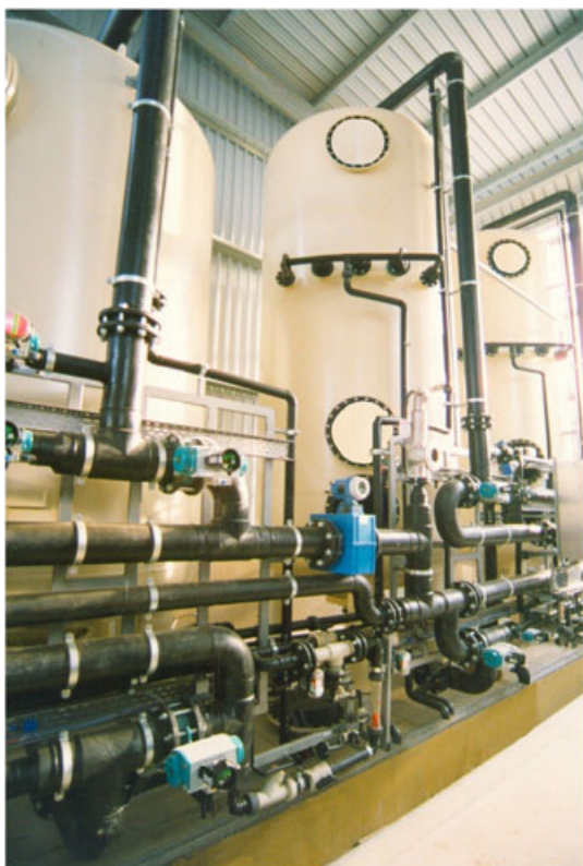
Figure 7. Cation exchanger in Africa, 140 \text{ m}^3 \text{ h}^{-1} (by EUWA).
