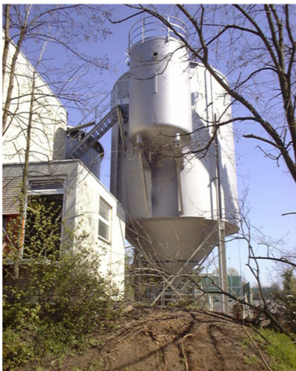
Figure 6. One-stage lime softening plant in Germany, 150 \text{ m}^3 \text{ h}^{-1} (by EUWA).
