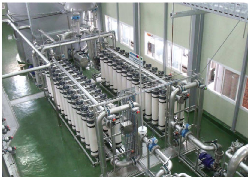
Figure 5. Ultrafiltration plant in Korea, output 270 \text{ m}^3 \text{ h}^{-1} , recovery 95% (by EUWA).
